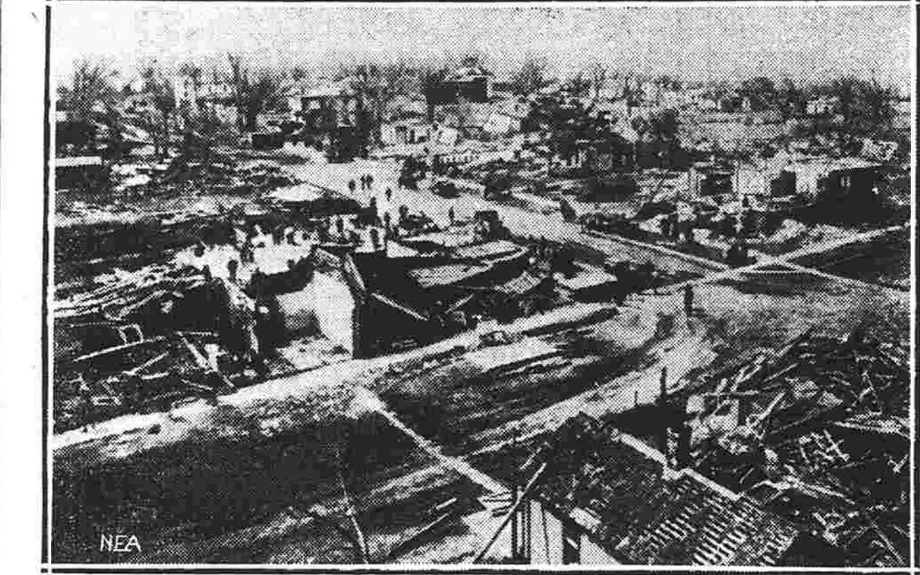
This remarkable telephoto picture shows the damage caused at Cornland, Ill., by a tornado that swept across the state, taking about 35 lives. Every building in the town was demolished or damaged, and people are shown seeking their belongings in the ruins. The picture was taken from the top of a badly damaged grain elevator.
